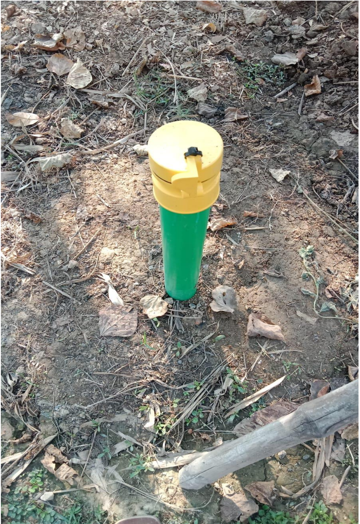
Fig: Barometric pressure meter after installation
